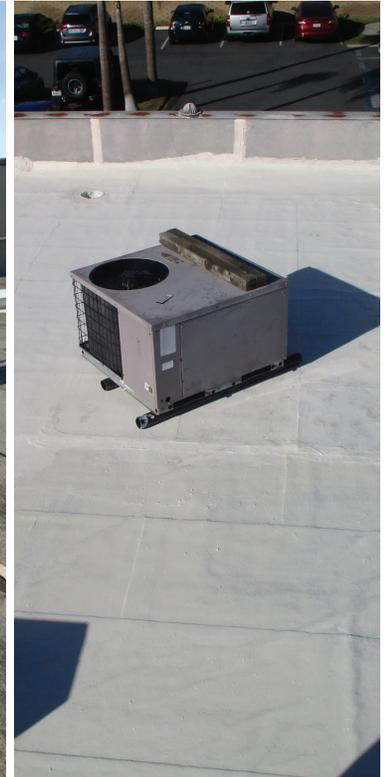
In this case, Ecodur also allowed for a lighter, more reflective top coat to be applied, thus greatly reducing the heat sink effect.
